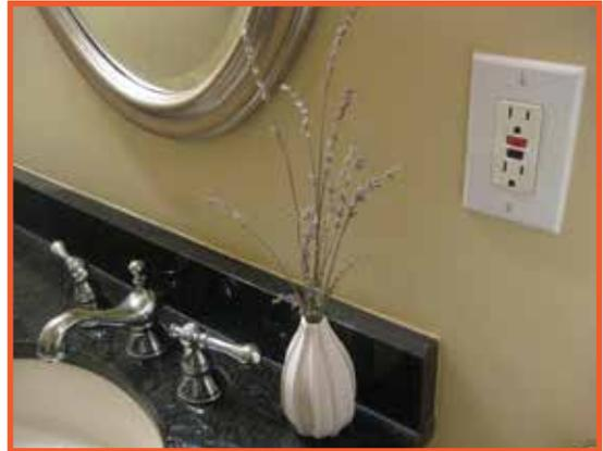
need to take is to test an item, such as a lamp, that visibly powers on when plugged in. Push the “reset” button to prepare the outlet then push the “test” button. Did your lamp turn off? If it did, the GFCI is working properly. Now, hit the “reset” button once again to power it back on. If your lamp did not power off, then you should contact a certified electrician to correct the problem.
